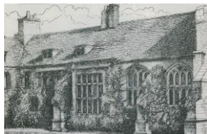
Corpus Christi - the Old Hall & part of the Old Court
